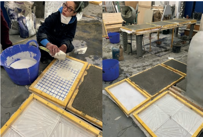
Casting of the panels. The image to the left shows the glass fibre mesh.
