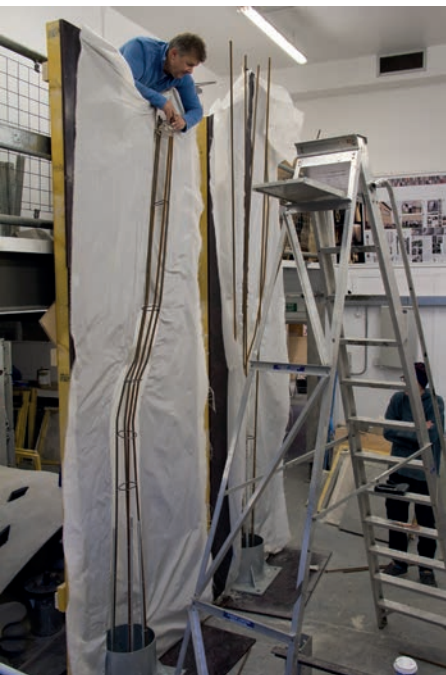
Fitting of the reinforcement with one half of each formwork erected.
